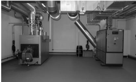
Fig. 4. Technical room of the combined heat and power plant (picture courtesy of Süwag Renewable Energy).
