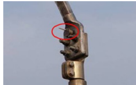
Fig. 2. Temperature sensor installation location
