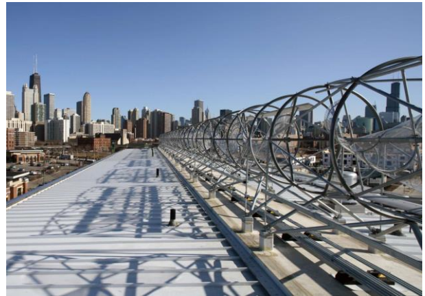
Fig. 12. Aerotecture turbines on Mercy Housing Lakefront rooftop – Chicago [10].
