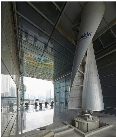
Fig. 11. Savonius VAWT inside Pearl River Tower – Guangzhou [9].
