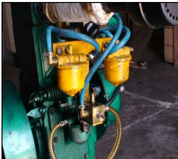
(a) Filter unit in position
