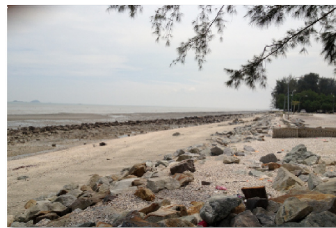
Fig. 1: Existing condition of coastal erosion in Pantai Remis, Kuala Selangor.
